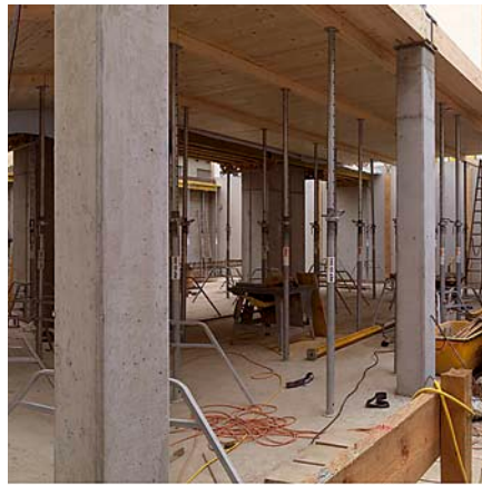
Pilari-palkkirunko on 320 x 360 mm liimapuuta. Maantasokerros on betonia. The building has a 320 x 360 mm glued column and beam frame. Ground floor is of concrete.
