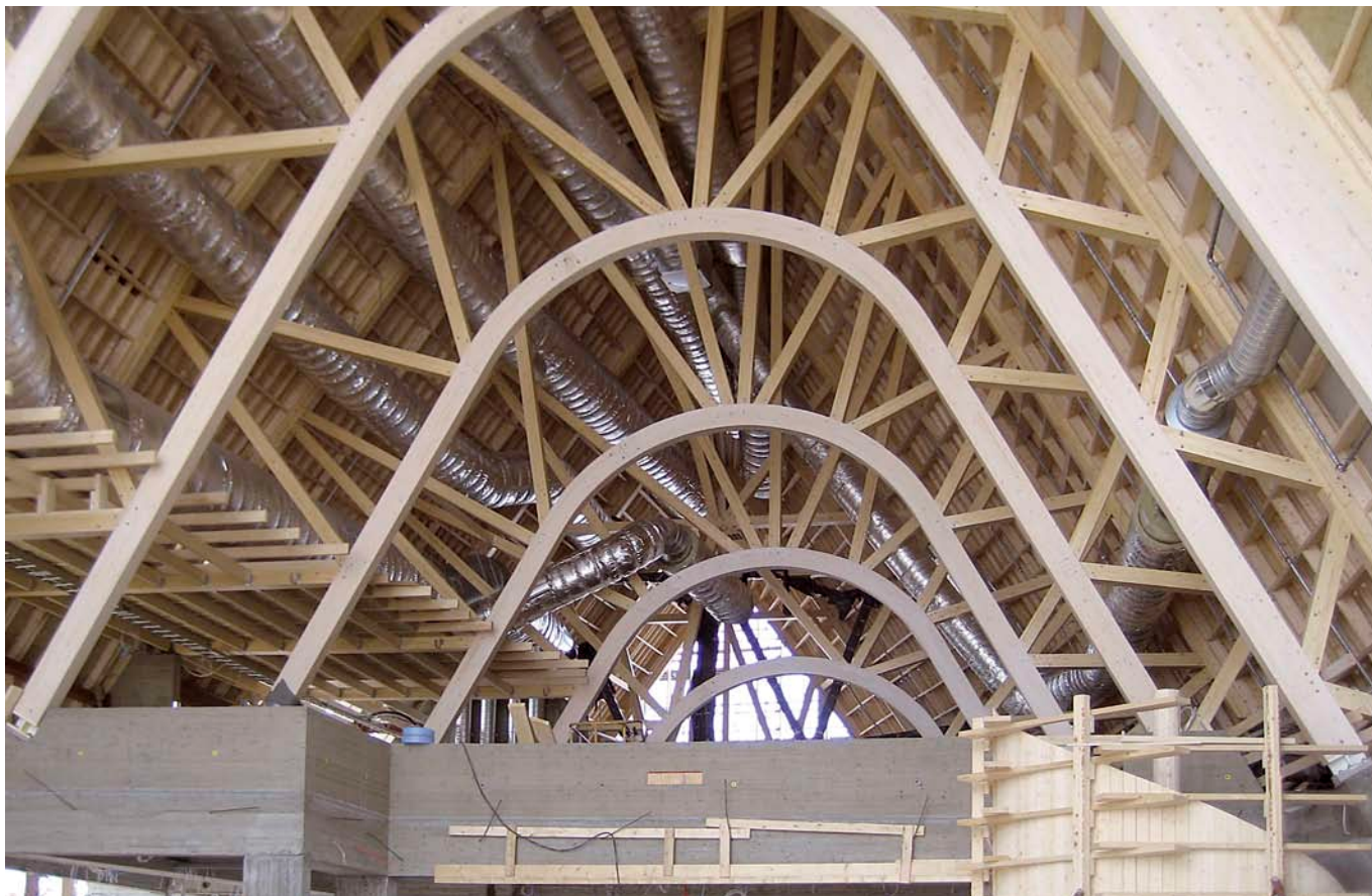
Verkkokuori koottiin paikalla kolmesta lamellista The gridshell was assembled and laminated together in-situ in three sections.
