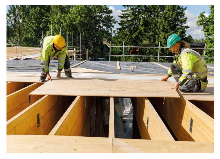
Roof structures can be designed in many different ways according to national building regulations and requirements. Strong and rigid spruce plywood is an excellent substrate for different roofing materials. Plywood panels can be also used as horizontal bracing for stabilizing the building. The light and dimensionally stable panels are easy to fit together and they can also be used as a safe working surface during the installation of the roofing.
