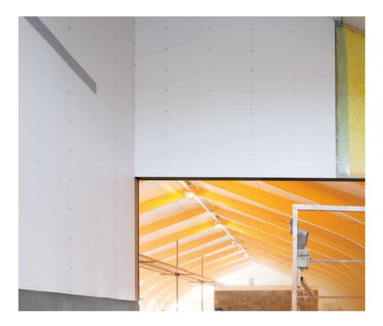
Metsä Wood Spruce Flex is a spruce plywood panel with a thermoplastic overlay. The technical advantages of spruce plywood combined with the thermoplastic overlay make Spruce Flex an excellent panel for various demanding interior applications. Spruce Flex panels have a smooth and light colour visual appearance, and an excellent impact and crack resistance. Surface is easy to clean with water and normal detergents.
