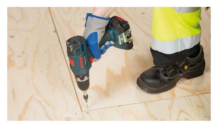
When fasteners are an essential part of the structural system, e.g. plywood is used as a bracing panel or plywood acts as a buckling support for studs, the boundary conditions according to EN 1995-1-1 should be taken into account.
