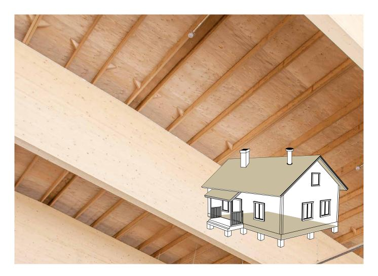
There is always a risk of mould growth on the surface of untreated wood products when they are located in high relative humidity conditions or in an unheated space where the humidity of the air may be high and condensation may occur from time to time. In end use applications, such as a roofing panel, Metsä Wood recommends the use of Metsä Wood Spruce MouldGuard plywood.
