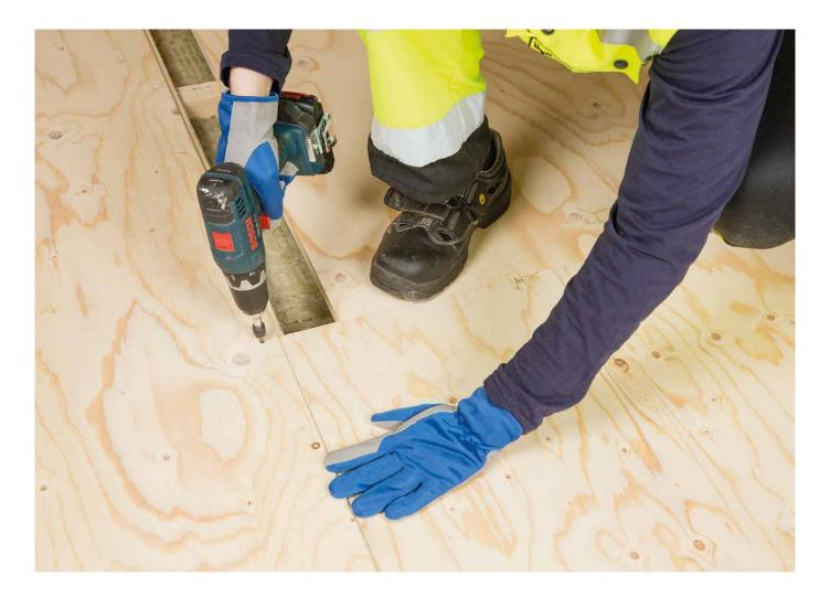
The strong and rigid spruce plywood flooring panels have a good load-bearing capacity. The smooth and uniform surface of the panels is an ideal foundation for parquet floors, carpets and floor tiles. Spruce plywood panels can also be used on their own as ready-made floors in warehouses and other similar applications. In particular, the small deflections of the panels make the use of longer spans possible, which in turn helps save the amount of construction material required.
