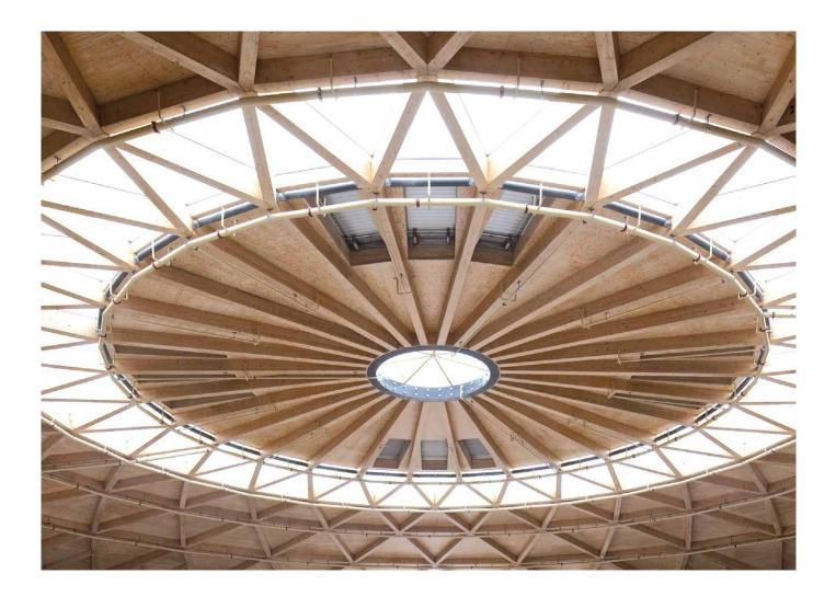
Metsä Wood Spruce is suitable for ceiling paneling as an assembly substrate for other interior lining materials or as a ready finished surface, giving a light, vivid and warm appearance for the room. Spruce panels can be coated with all standard stains, lacquers and paints suitable for wood products.
