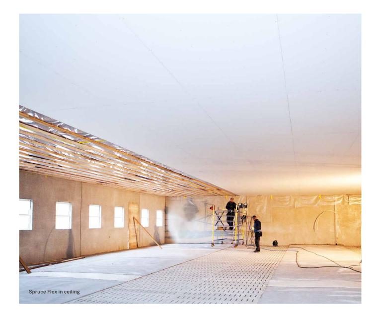
Ceiling panels can be installed in two ways: panels can be fastened under the rafters/joists or panels can be fastened on top of rafters when both rafters and ceiling panels are visible. Panels installed under the rafters/joists should be fastened using threaded nails or screws according to EN 14592. Smooth nails are not allowed.
