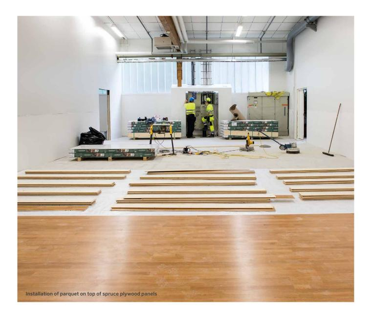
Metsä Wood Spruce plywood is a strong, rigid and durable flooring panel, well suited for use as an assembly substrate for different surface materials, or as a ready-made floor panel.
