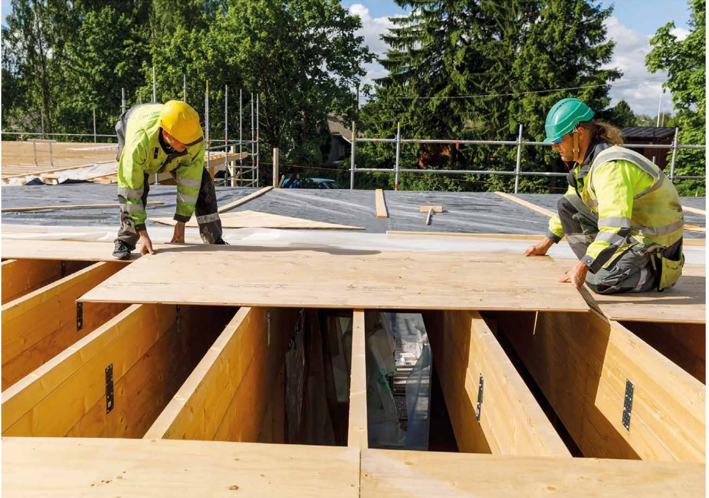
Roof structures can be designed in many different ways according to national building regulations and requirements. Strong and rigid spruce plywood is an excellent substrate for different roofing materials. Plywood panels can be also used as horizontal bracing for stabilizing the building. The light and dimensionally stable panels are easy to fit together and they can also be used as a safe working surface during the installation of the roofing.
