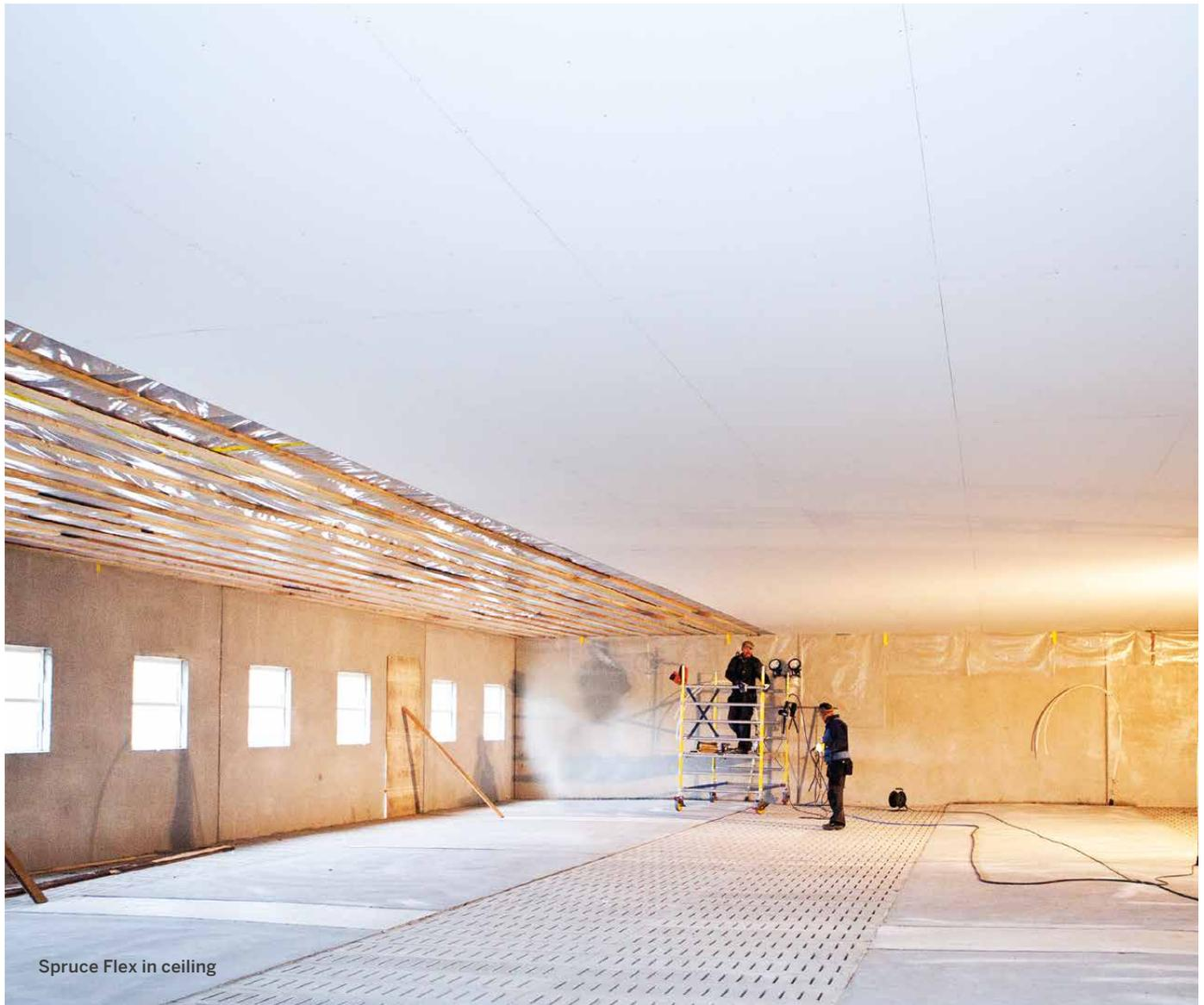
Ceiling panels can be installed in two ways: panels can be fastened under the rafters/joists or panels can be fastened on top of rafters when both rafters and ceiling panels are visible. Panels installed under the rafters/joists should be fastened using threaded nails or screws according to EN 14592. Smooth nails are not allowed.
