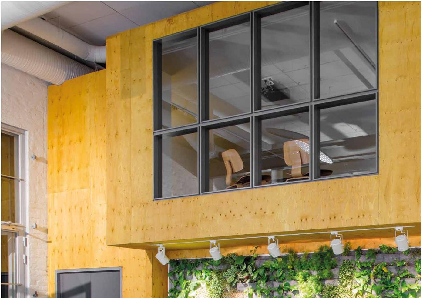
Spruce FireResist is suitable for use as wall, floor and ceiling panel and it offers a visible wood surface. Additional coatings are not recommended for Metsä Wood Spruce FireResist as coatings might affect the fire performance of the plywood. The compatibility of the surface treatment should be confirmed from the paint or varnish supplier.
