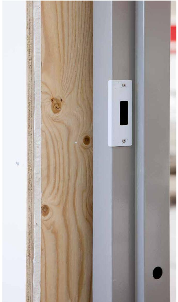
Spruce Flex is used to protect gypsum board wall
