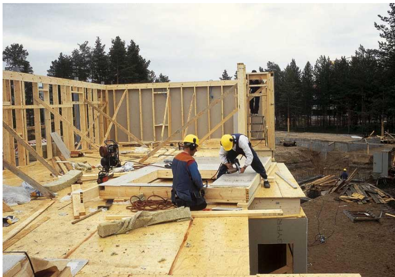
Figure 4. Typical platform-frame construction in Oulu in 1996.
